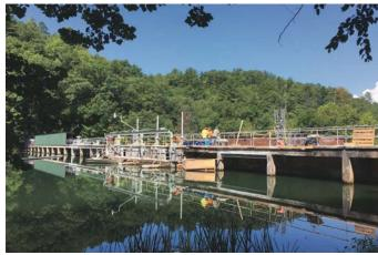
the buttress, giving the carbon fiberced polymer (CFRP) a "mechanical " CFRP was then installed over the anchors and wrapped over the four sides of the buttress. Upon completion, two coats of Class 5 coating were applied. New forms where installed along the sides of the walkway as well as the sides of the beams and archway. The archway was placed from the top
