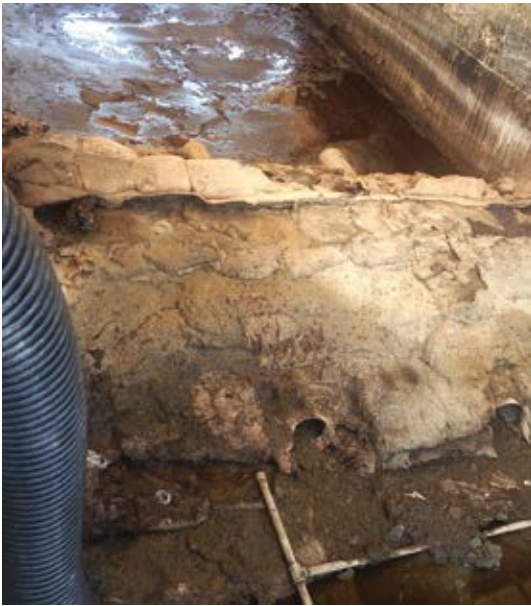
Condition of dike once Mix Box was drained
