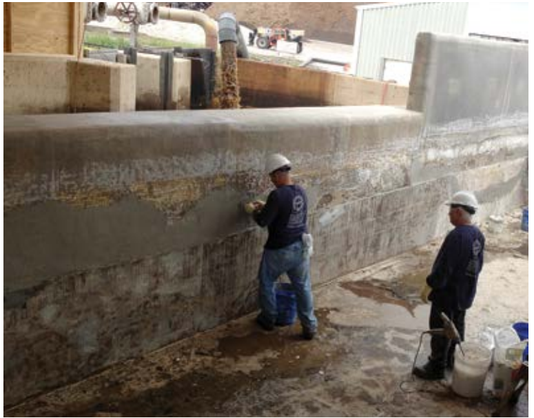
Surface preparation underway
