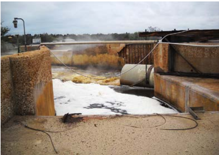
New FRP dike installed
