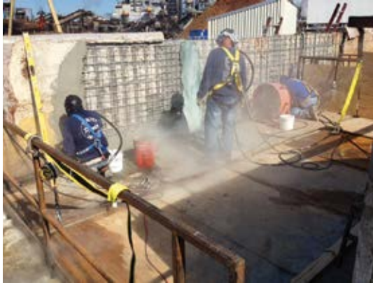
Columns are installed first to receive formwork for wall
