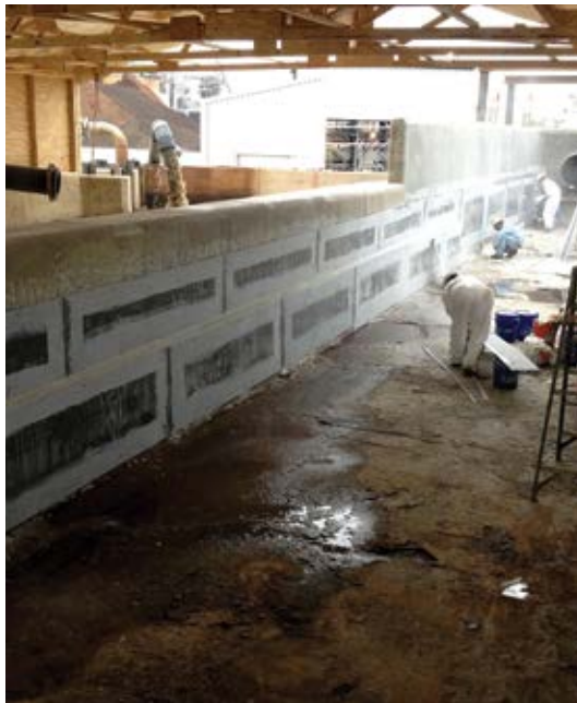
FRP panels prepared to be welded to each other
