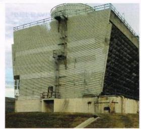
uilt in 1976, this 255 x 68 in. (77.7 x 20.7 m) cooling tower is divided into six different chambers. The "overflow channel" is 8 ft (2.4 m) wide x 255 ft (77.7 m) long. This is where most of the concrete repairs took place. The scope of the work included designing the repair and strengthening system of the walkway. This area is similar to a bridge piling. With advanced corrosion and concrete deterioration, operation of the facility came dangerously close to forcing a shutdown.
